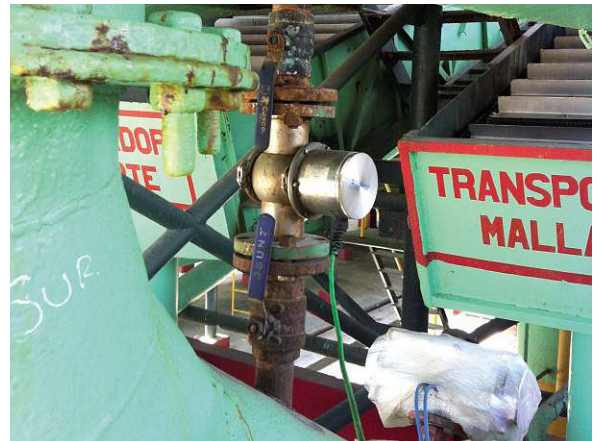
PhaseGuard in bypass installation DN100
