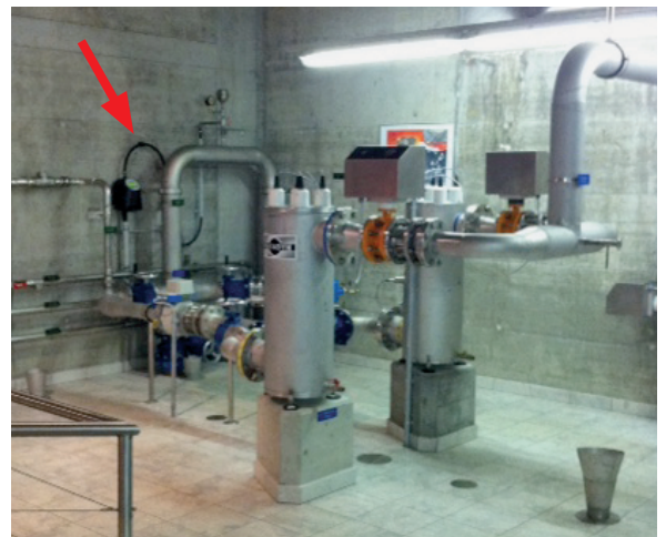
UV reactors with AquaScat WTM before/after disinfection
