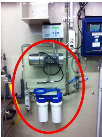
Picture: ColorPlus Bypass in raw water with filtration of sample
