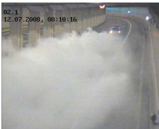
From experience it is known that the linear fire alarm cables normally already installed in the tunnel cannot detect such incidents. Such systems only react once there is an open fire which causes a change in the temperature. Neither are video detection systems able to cope with such situations as too many false alarms are triggered due to light reflexions from windscreens, change of contrast, etc.
