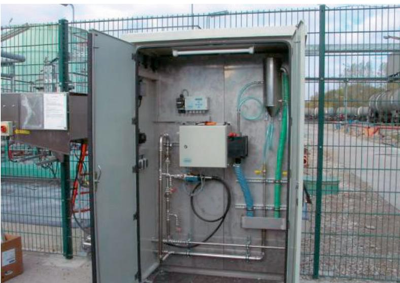
*Oil traces monitoring of collected waste water from a fuel storage area*
