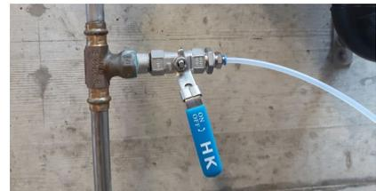
**Figure 5:** Simple control of the required water flow rate of 200 to 400 ml/min when continuously measuring with the BactoSense
