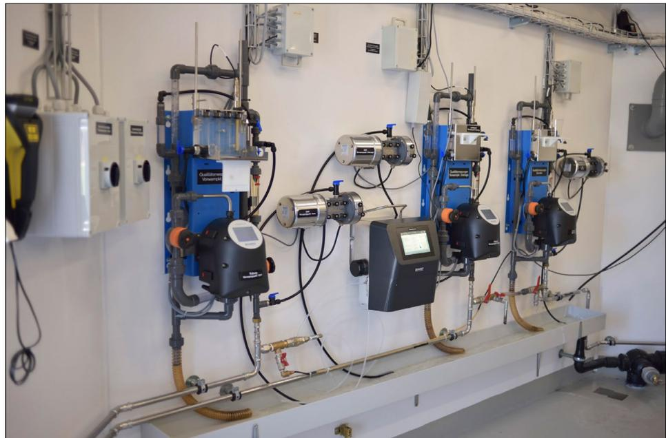
Figure 2: BactoSense installed in a groundwater well
